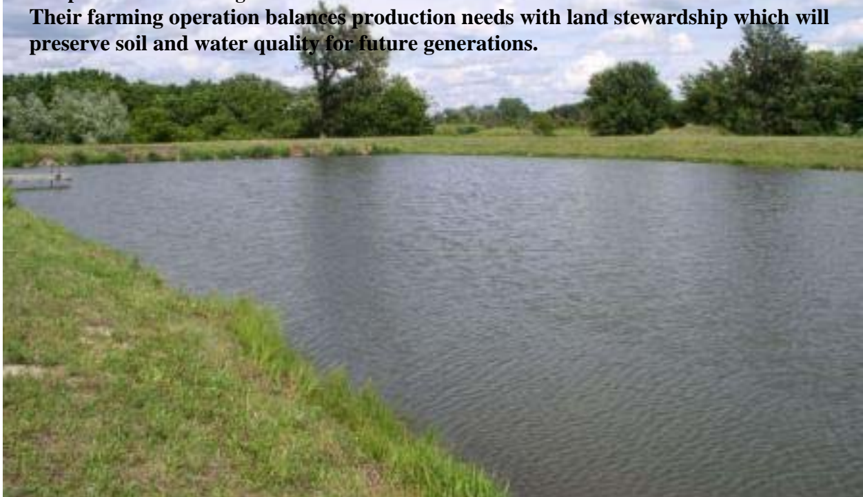
Grade Stabilization Structure
